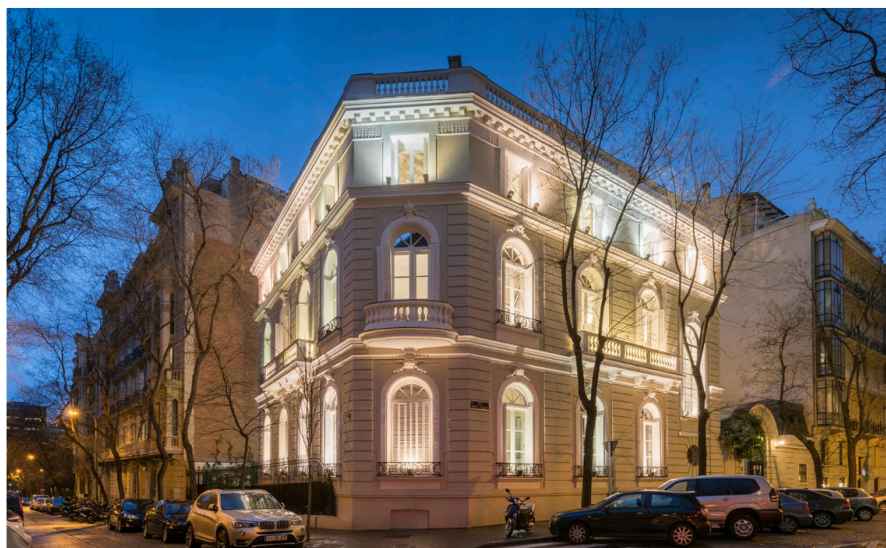
Exterior of the Norman Foster Foundation headquarters in Madrid
