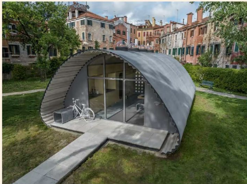
A prototype of the new shelter, installed in Venice © Chiara Becattini
